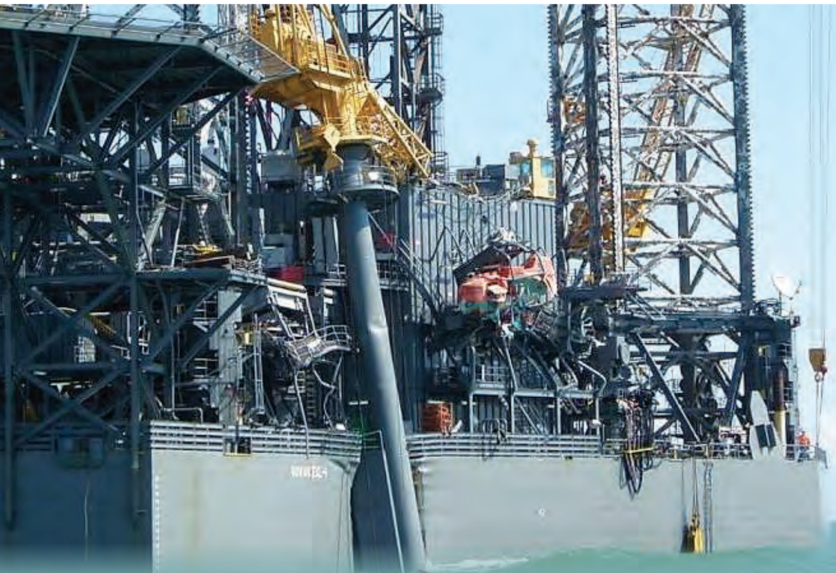
The extensive damage to the port side of the Rowan EXL I , including its destroyed survival crafts (orange-colored) near the center of the photo. Photo provided by the Coast Guard.
