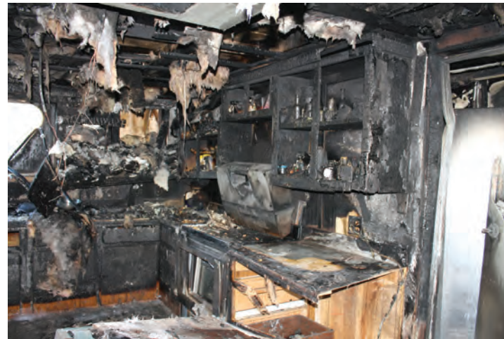
Figure 47: Fire damage to the towing vessel San Gabriel galley located on the main deck. PHOTO BY COAST GUARD
