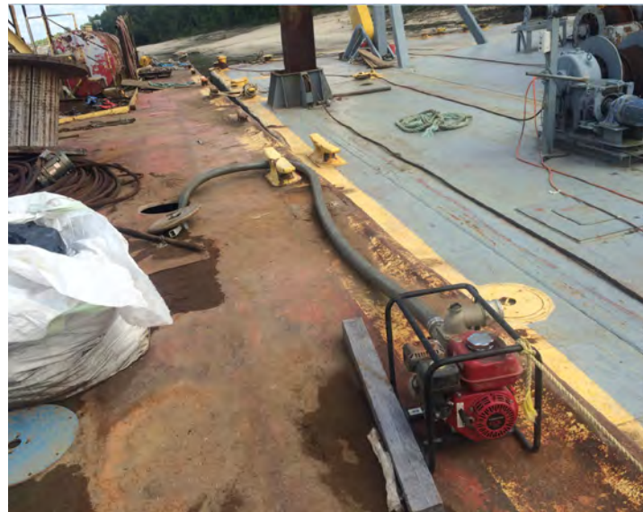
Figure 53: Portable pump and hose rigged to dewater a void on a similar deck barge.
