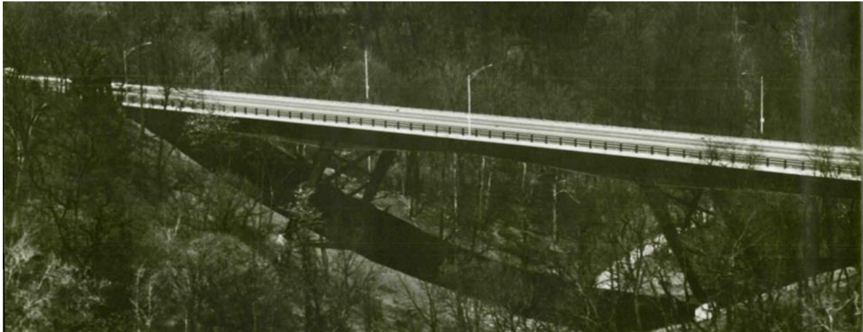
Figure 5. 1973 Fern Hollow Bridge (Source: National Steel Bridge Alliance, 1974 Prize Bridges ).
