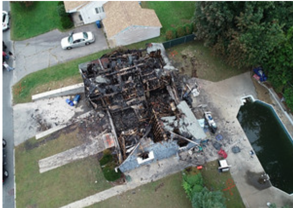
Figure 7 An aerial view of a burned-out home impacted by natural gas explosion and fire in Merrimack Valley, Massachusetts. The photo was captured by a drone operated by an NTSB investigator to document the damaged caused by the explosions and fires.
