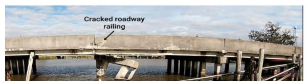
**Figure 10** Damage to the Route 182 bridge, which was struck by towing vessel *Miss Mollye D* between Morgan City and Amelia, Louisiana, on December 23, 2021. The NTSB issued Marine Investigation Report 23/04 on February 9, 2023, detailing our investigation of the collision. (Source: US Coast Guard).
