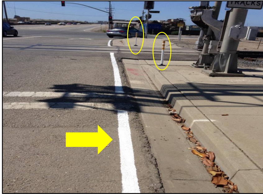
Figure 11. Interim improvements at grade crossing: 4-inch-wide solid white edge line and two white tubular markers installed postcrash.
