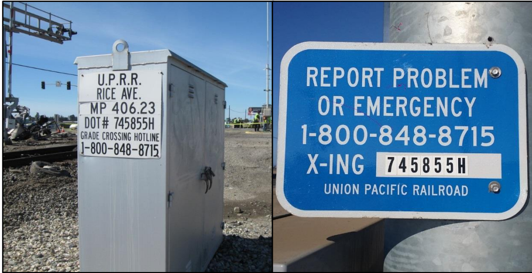
Figure 6. Signal bungalow near South Rice Avenue grade crossing, and one of two blue signs mounted on the cantilever signal masts, showing emergency telephone and grade crossing numbers.
