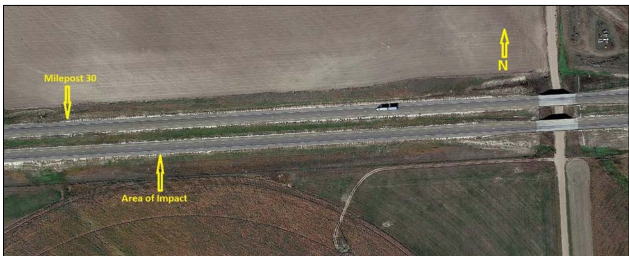
Figure 2. Aerial view of crash location near milepost 30 eastbound on US-70, indicating area of impact. (Source: Google Earth modified)
