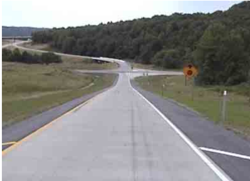
Figure 11. Exit ramp from I-540 south to SH-282.
