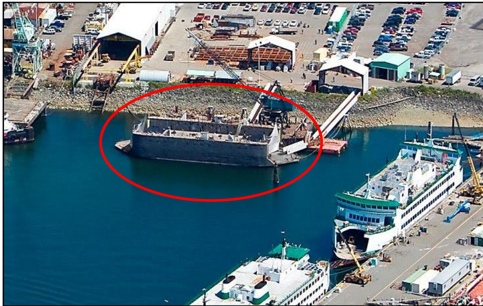
Aerial View of Dry Dock #3 at Port of Everett. (Photo by Vigor Industrial, LLC)
