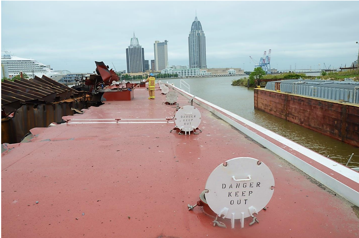
Open tank hatches on Kirby 28194 , photographed after the accident, through which flammable vapors were being vented. Undamaged barge DM 976 can be seen on the right. (Photo by the Coast Guard)
