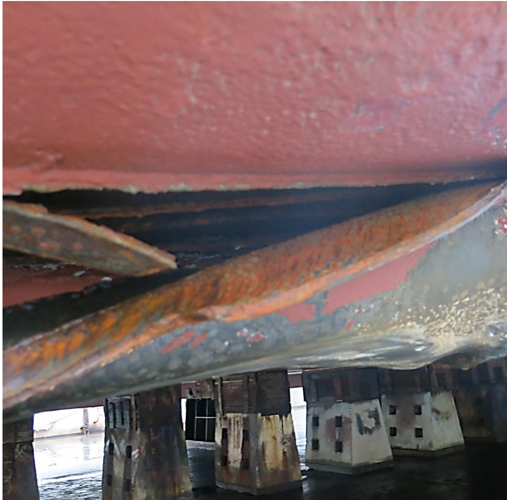
Breached hull on the Gordon Jensen 's port side.
