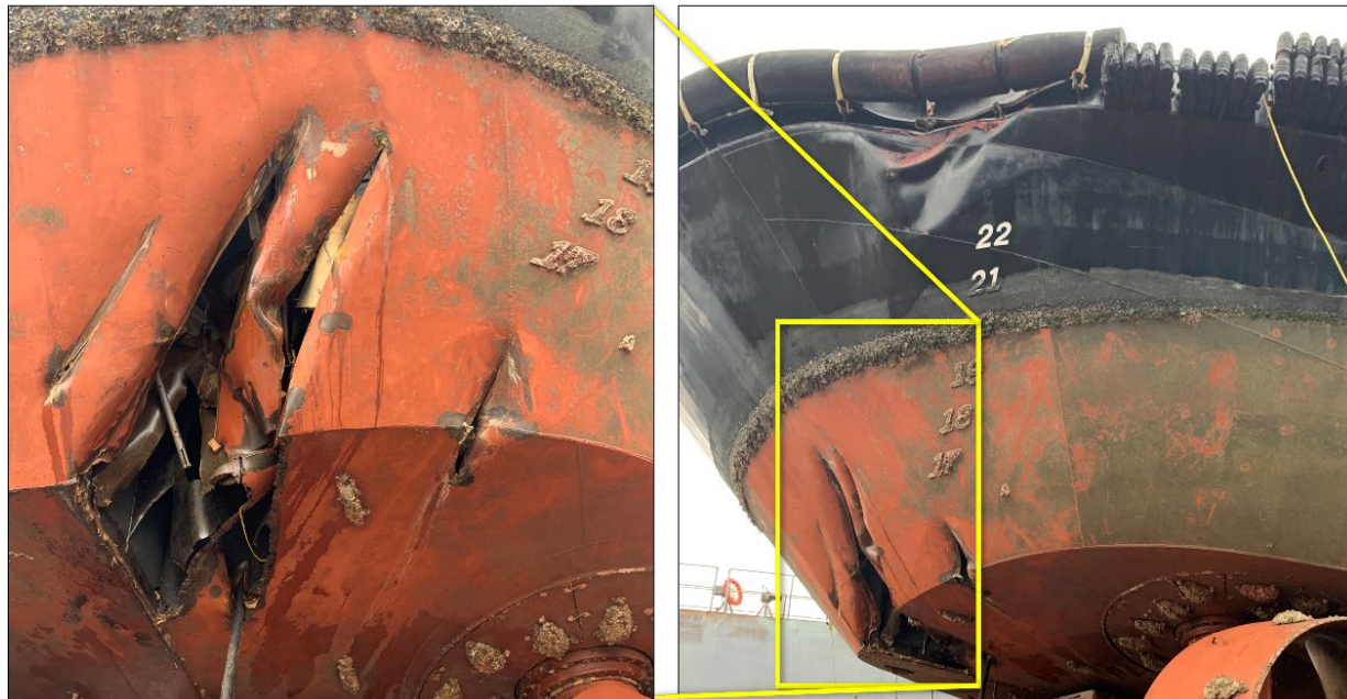
Figure 5. Damage to Mark E Kuebler stern hull and fendering system from the Nisalah propeller.
