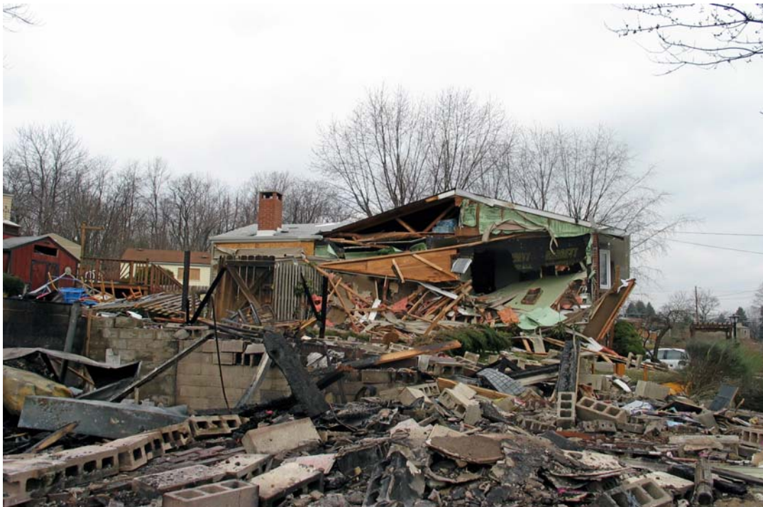
Figure 1. Damage to 171 Mardi Gras Drive.
