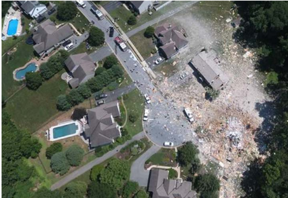
Figure 1. Debris field at cul-de-sac area where explosion occurred.
