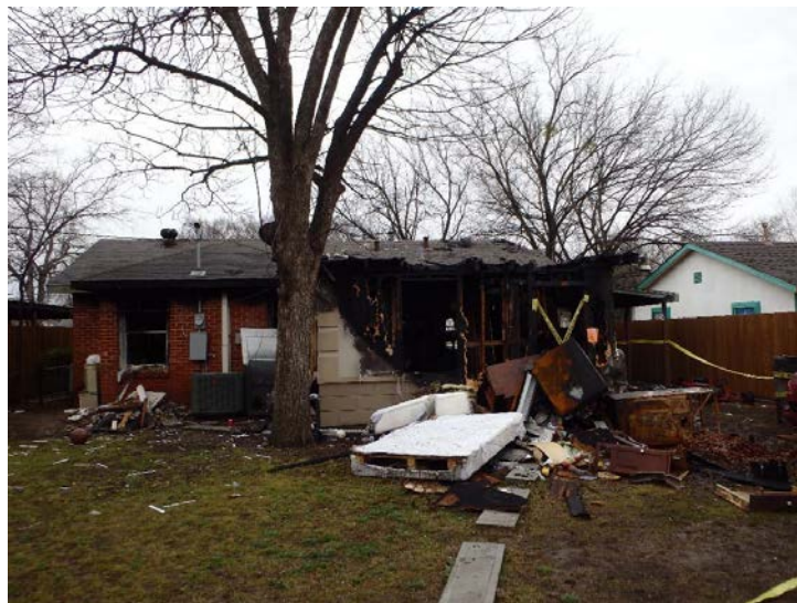
Figure 4. Post-fire view of the residence at 3515 Durango Drive.
