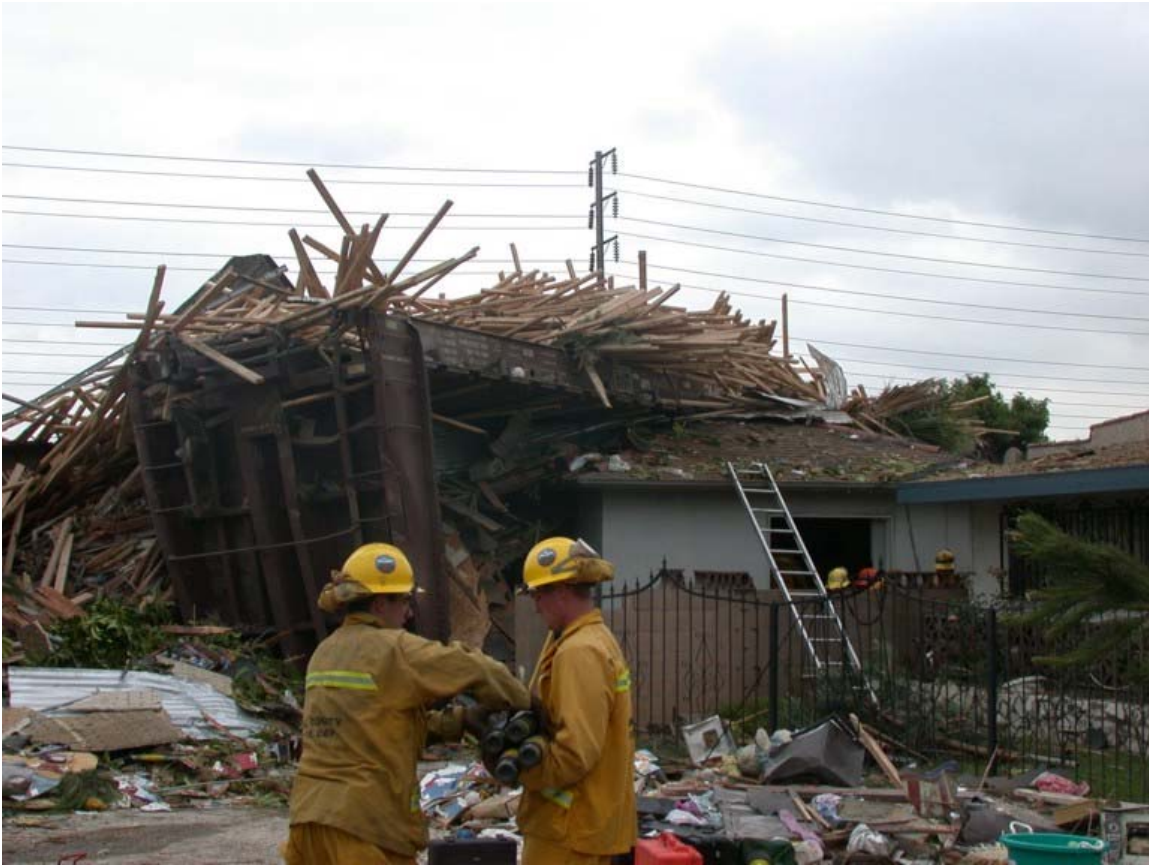
Figure 2. One of the eight residences struck by derailed equipment.
