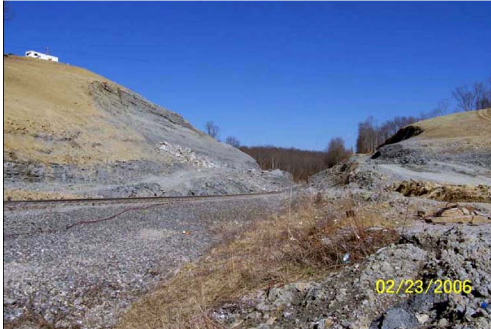
Figure 2. The track after removal of hill and Eagle Tunnel No. 3.
