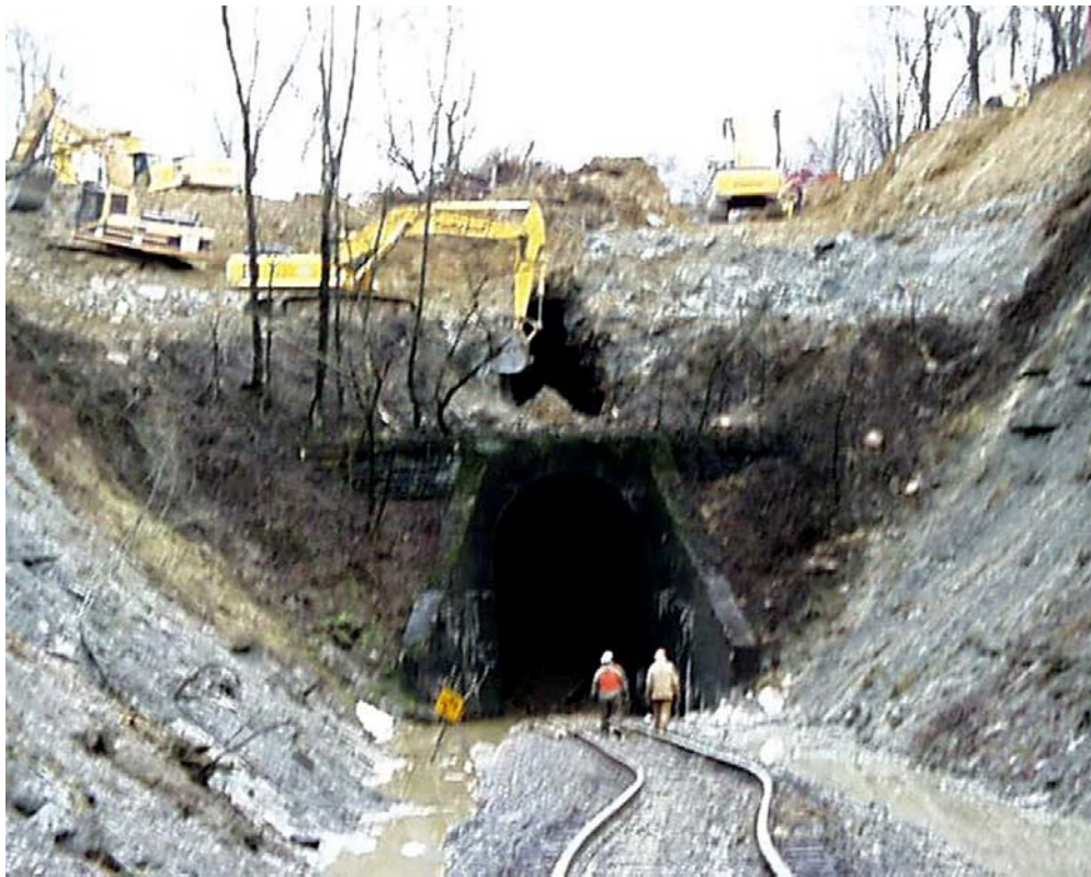
Figure 1. Excavation of Eagle Tunnel No. 3. (Track misalignment caused by derailment.)
