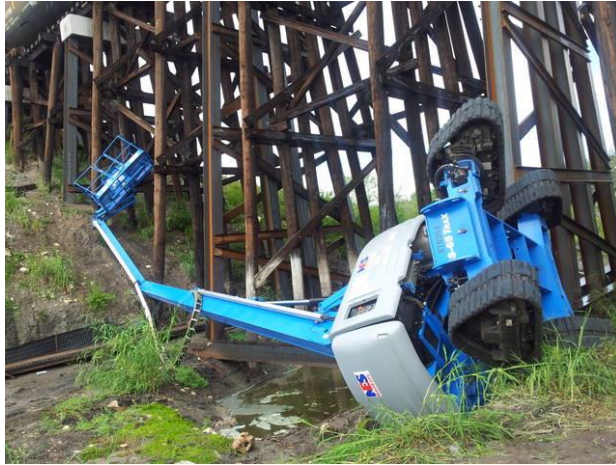
Figure 3. The overturned S-60 Trax aerial lift vehicle.
