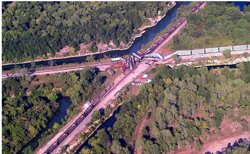
Figure 1. The accident site.
