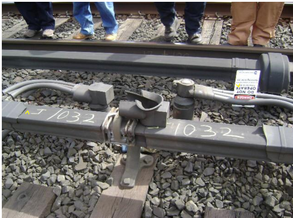
Figure 3. Jumper inserted in receptacle and considered “closed.”
