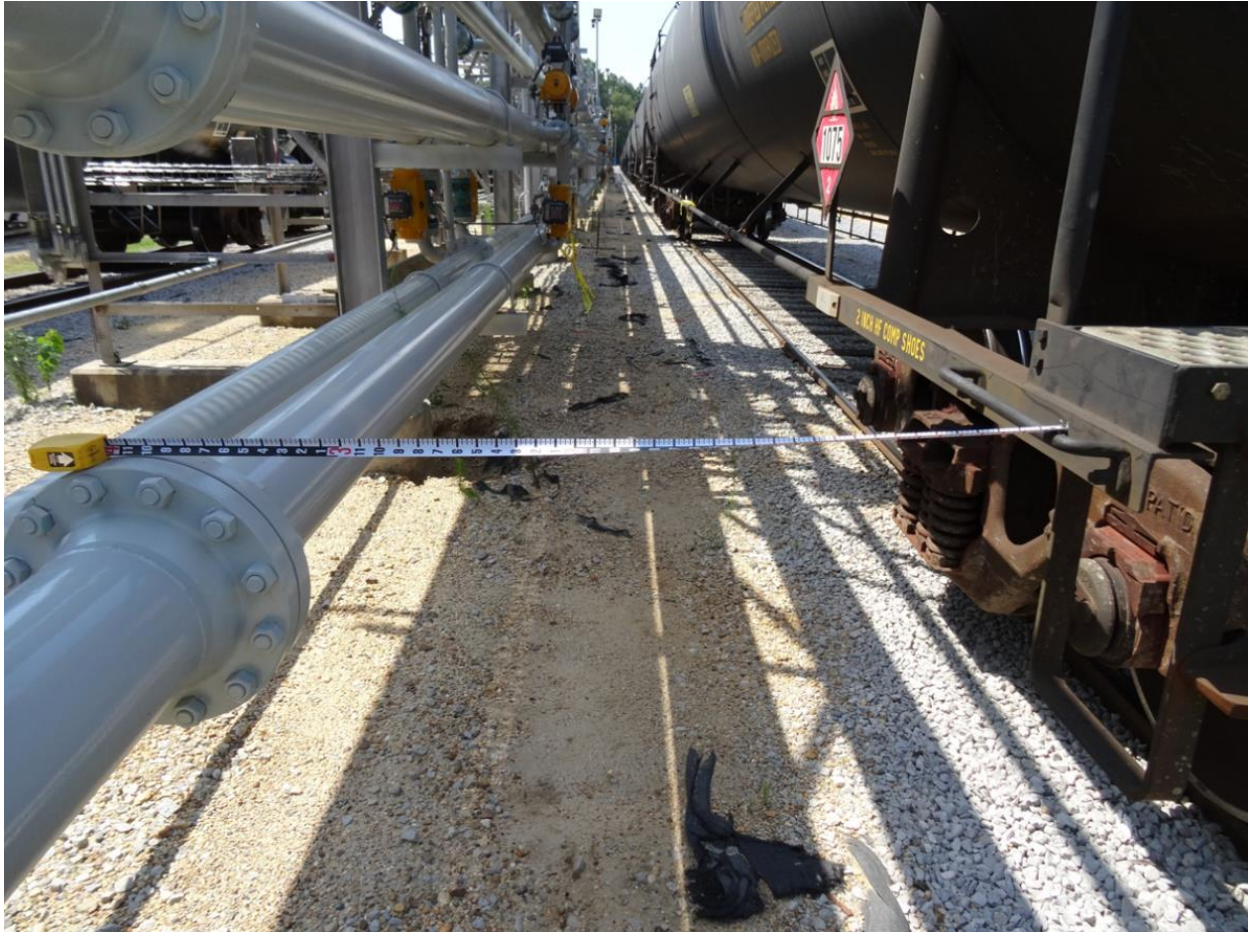
Figure 2. Path between the tank cars and unloading rack in the H 82 gas plant.
