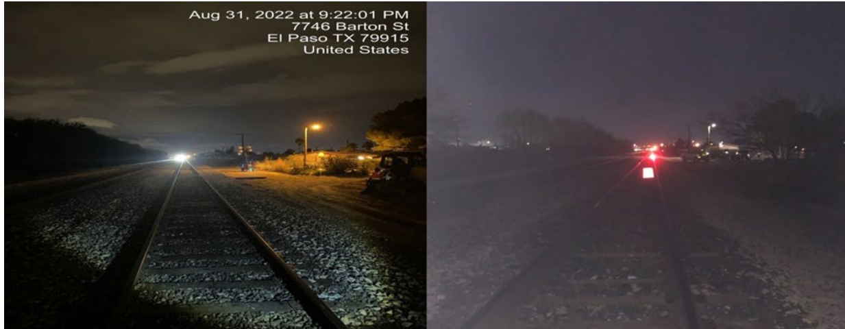
Figure 5. Derail with a sign on the night of the accident (left), derail with the reflectorized flag and red light after rule changes (right). (Left image: courtesy of UP; right image: courtesy of the International Association of Sheet Metal, Air, Rail and Transportation Workers.)
