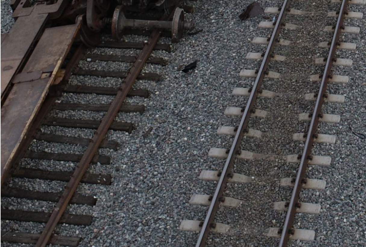
Figure 5. Rail conditions on Bertram siding ( left ) and main track ( right ).
