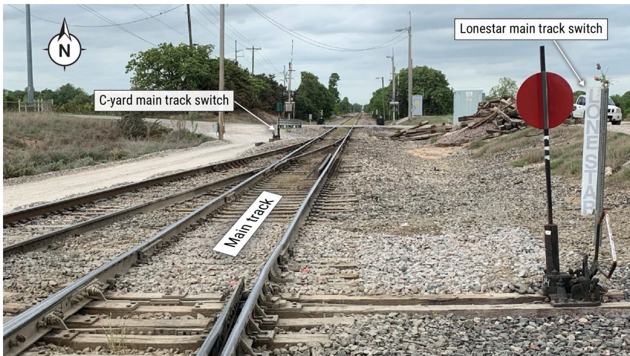
Figure 2. Photograph of the main track, the C-yard main track switch, and the Lonestar main track switch. (Courtesy of UP.)
