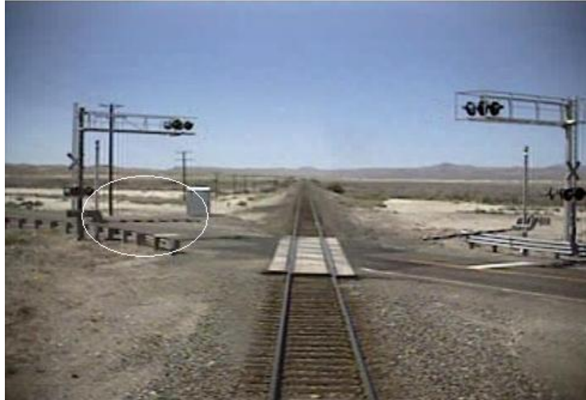
Figure 19. Video frame capture from Amtrak train no. 5 at 11:19:24 a.m., about 4 seconds prior to accident truck collision, showing crossing gate arms in descended position on northbound (circled) and southbound sides of US 95. At point of image capture, accident truck is approaching grade crossing but outside video camera field of view.
