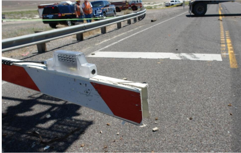
Figure 17. Photograph showing damage to tip of crossing gate arm in northbound lane of US 95. (Courtesy of Nevada Highway Patrol)
