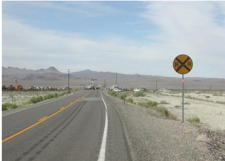
Figure 21. Photograph showing advance warning sign on right side of roadway, with pavement marking painted on northbound lane of US 95 about 140 feet beyond sign. (Tire marks in advance of pavement marking were determined not to have originated from accident truck.)
