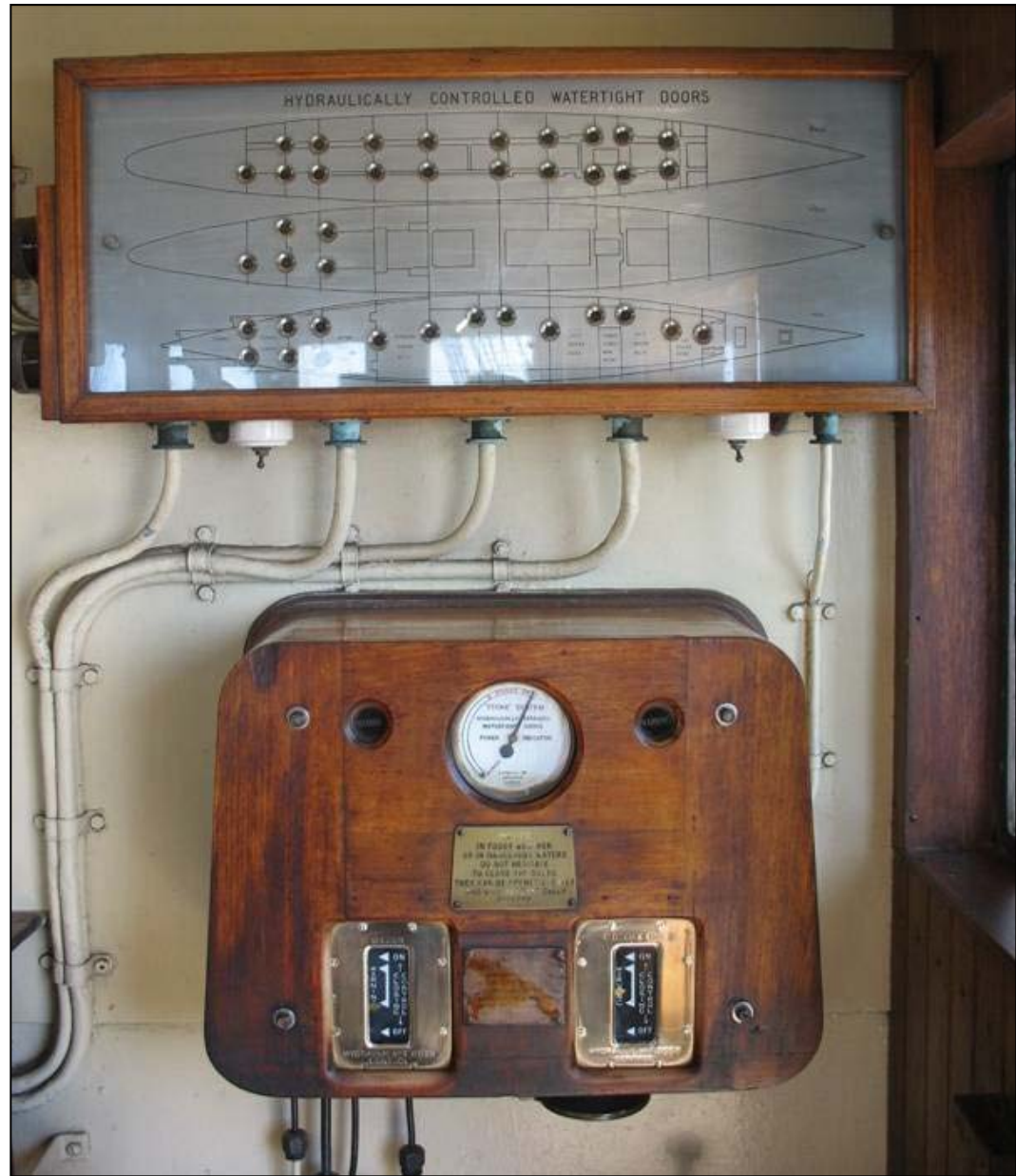
Watertight doors indicator and control mechanism
